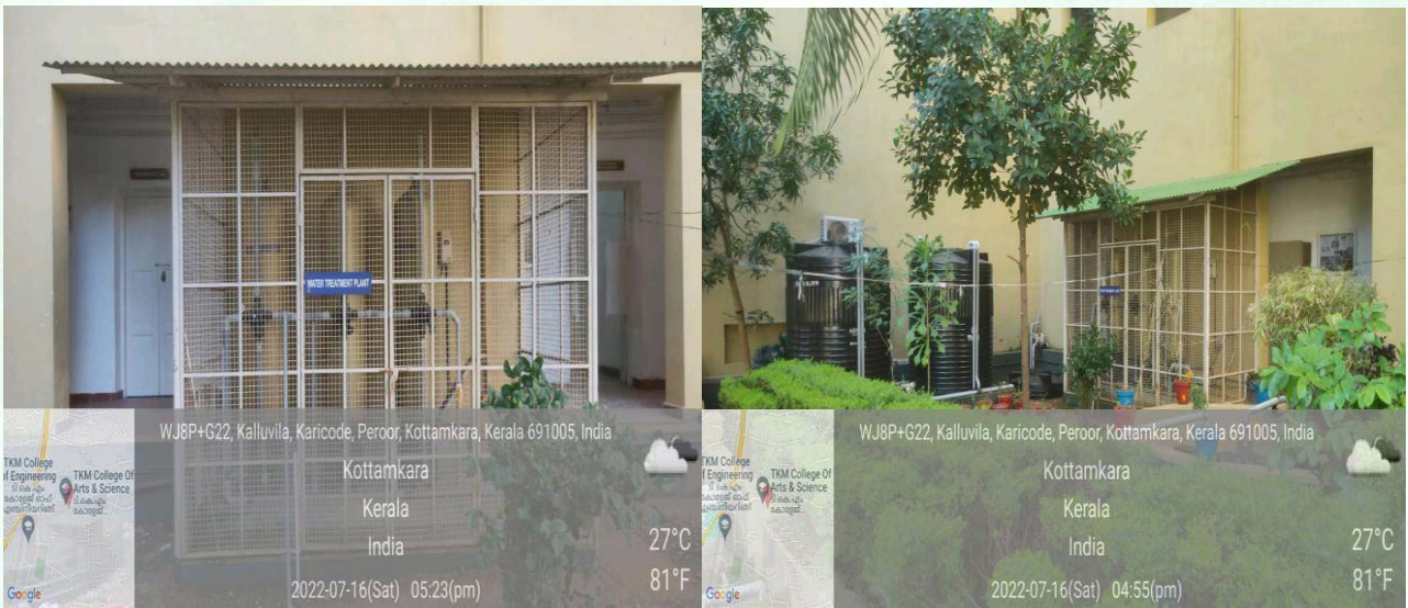
Water conservation and management Tanks in our campus
